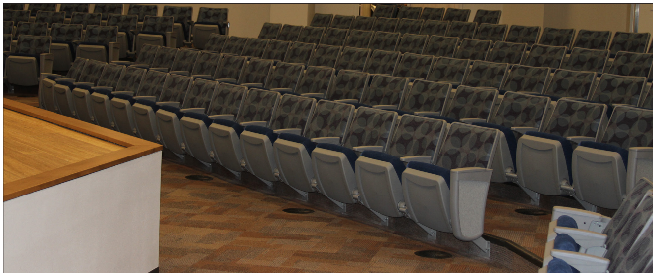
Figure 11. TAF-R diffusers in an under seat application
