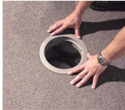
Figure 8. Trim ring installation
