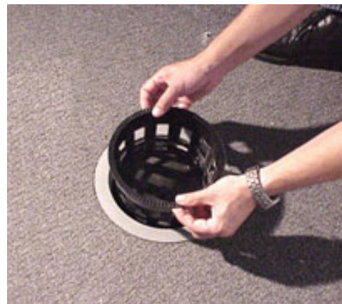
Figure 9. Basket installation
