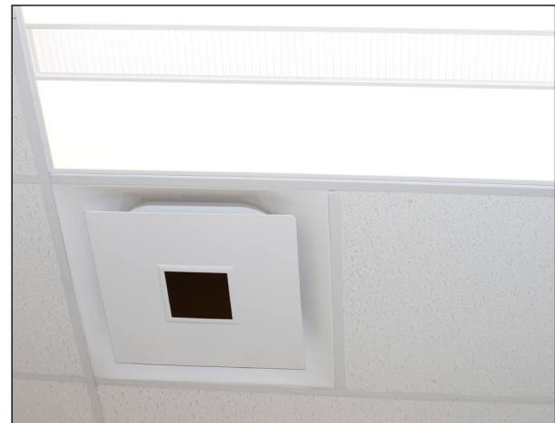
Helios VAV digital solar-powered diffuser installed in the ceiling of an office building
