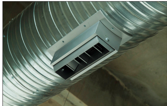
Installation images of the S-DL drum louvers installed in an open ceiling office environment
