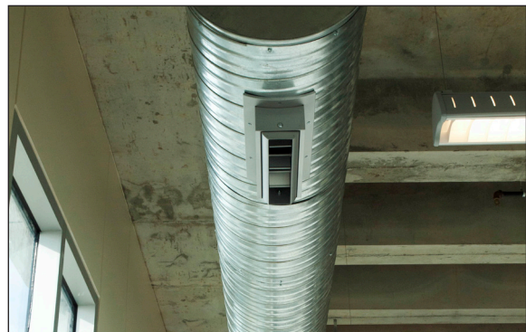
Installation images of the S-DL drum louvers installed in an open ceiling office environment
