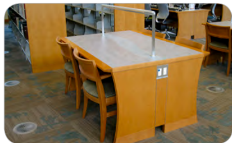
TAF-R diffusers with swirl face installed in the floor of a library
