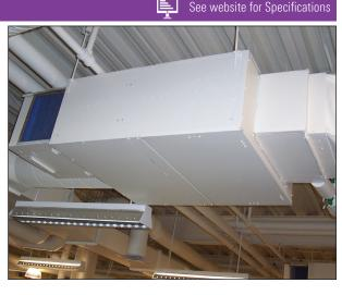
The Titus TFS-F Fantom IQ™ terminal unit installed in an open ceiling environment of a corporate office
