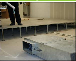
LHK terminal unit installed in an underfloor application
