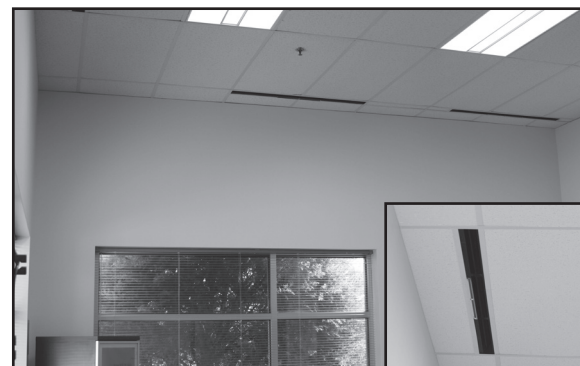
Below: EOS Master-Drone (DR) configuration installed in an office environment along the perimeter
