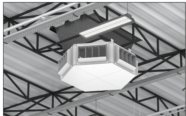
TVM-6 Typical installation
