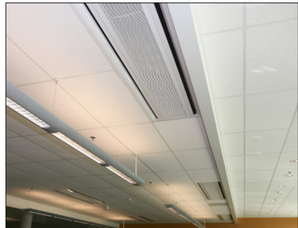
CBAL2 installed in the ceiling of a school
