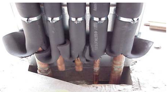
Cut insulation neatly in vertical manner
