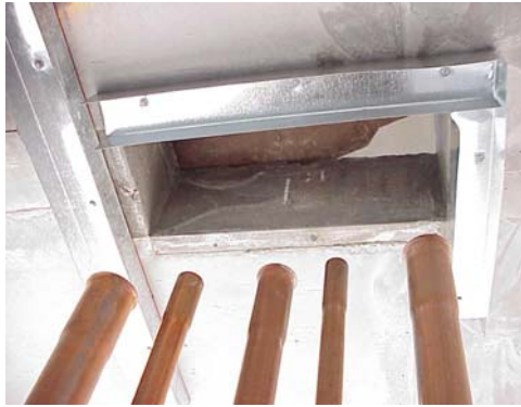
Top of riser incorporating female fitting
