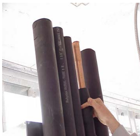
Push insulation back before soldering
