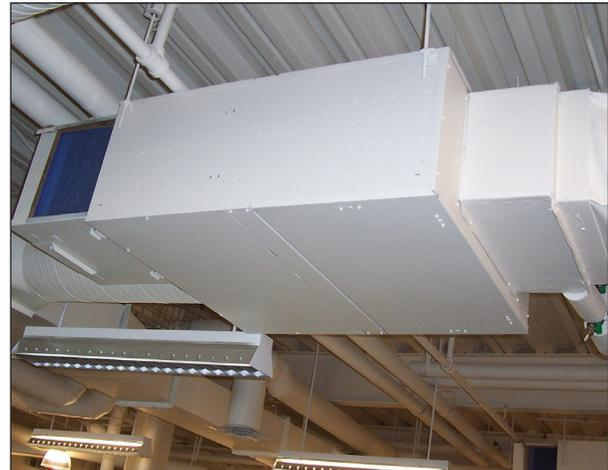
The Titus TFS-F Fantom IQ™ terminal unit installed in an open ceiling environment of a corporate office
